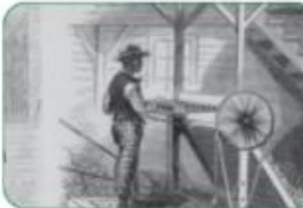
The cotton gin had a device that pulled the cotton through wire teeth. The seeds were caught by the teeth and pulled from the cotton fibres. By solving the tedious and time-consuming problem of the cotton seeds, the cotton gin made cotton extremely profitable.
