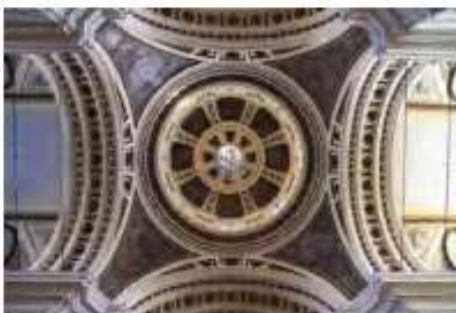
Figure 13 Spaces between arches set in a square to support a dome are called spandrels and are often decorative. Some features in organisms might be like spandrels, a consequence of another adaptation.
