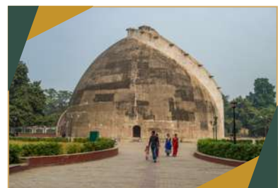
Figure 37 A granary to store grain built by the British East
