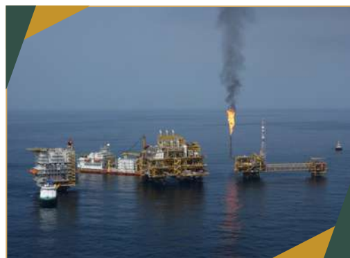
Figure 105 Nigerian Offshore Oil Platform
