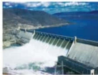
Figure 3 Hydroelectric energy plants use the gravitational potential energy stored in water to produce electricity.
