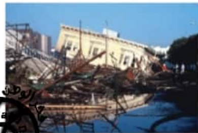
Figure 8 The seismic energy of a large earthquake caused severe damage to this building in San Francisco, California. In some locations, newly constructed homes and buildings are built to withstand many earthquakes.
